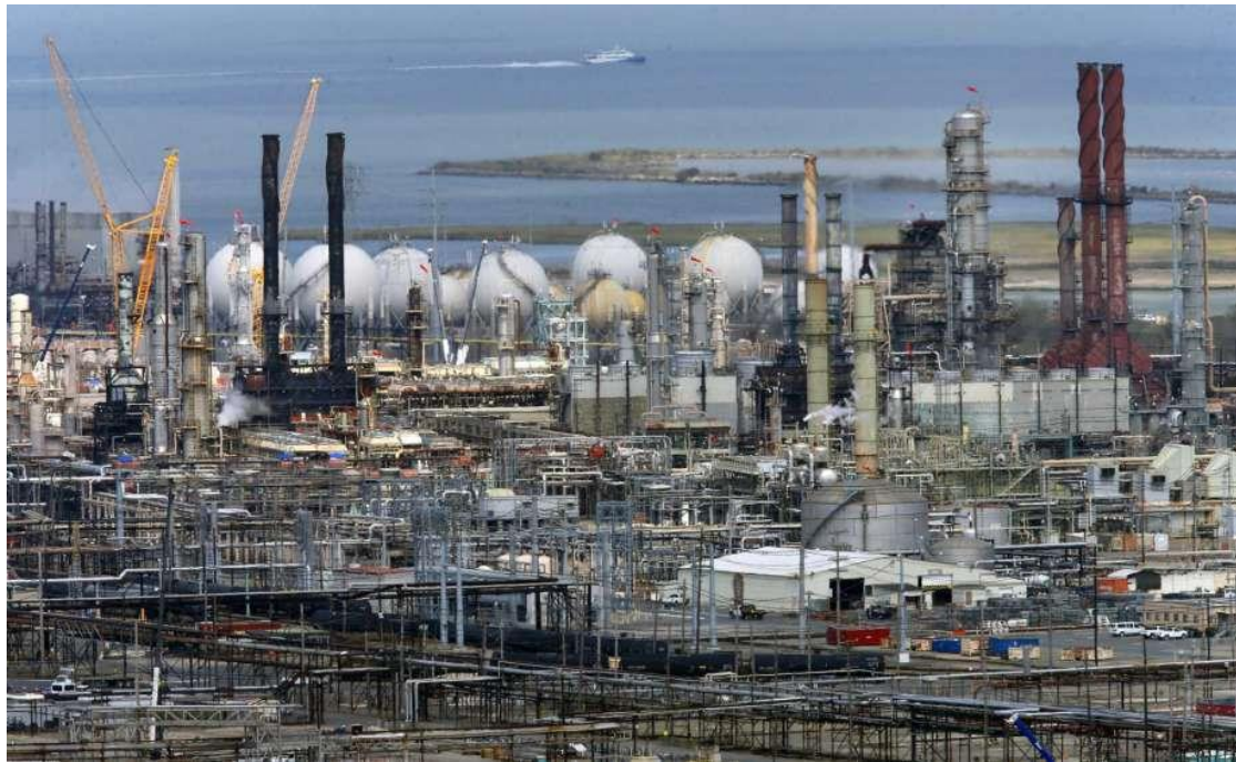
Chevron refinery, Houston
